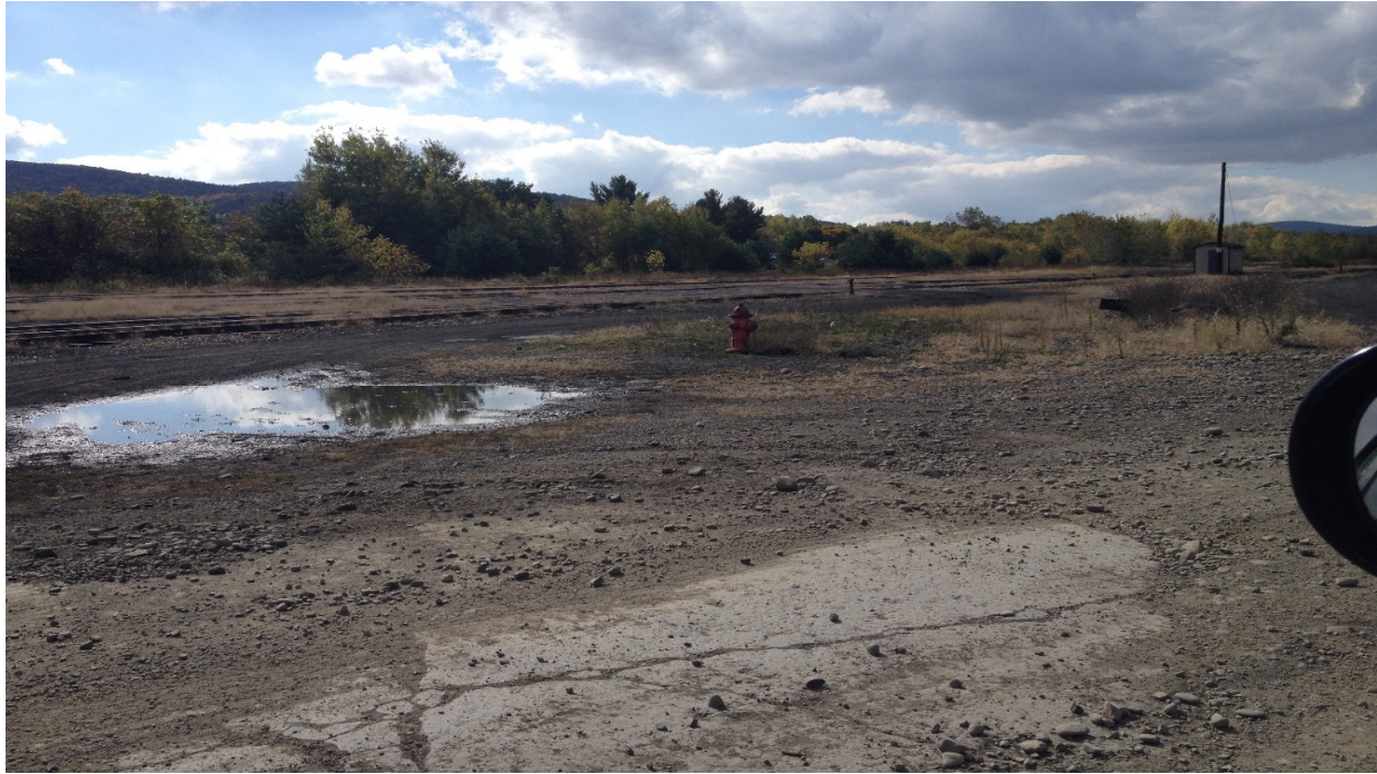
Intersection of Fonda Ave and Fonda Ave Extension looking southwesterly.
