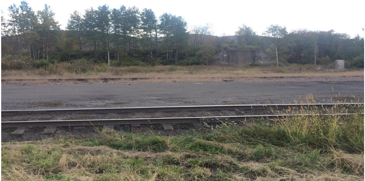
Roundhouse Road looking southerly across railyard at existing abutment.
