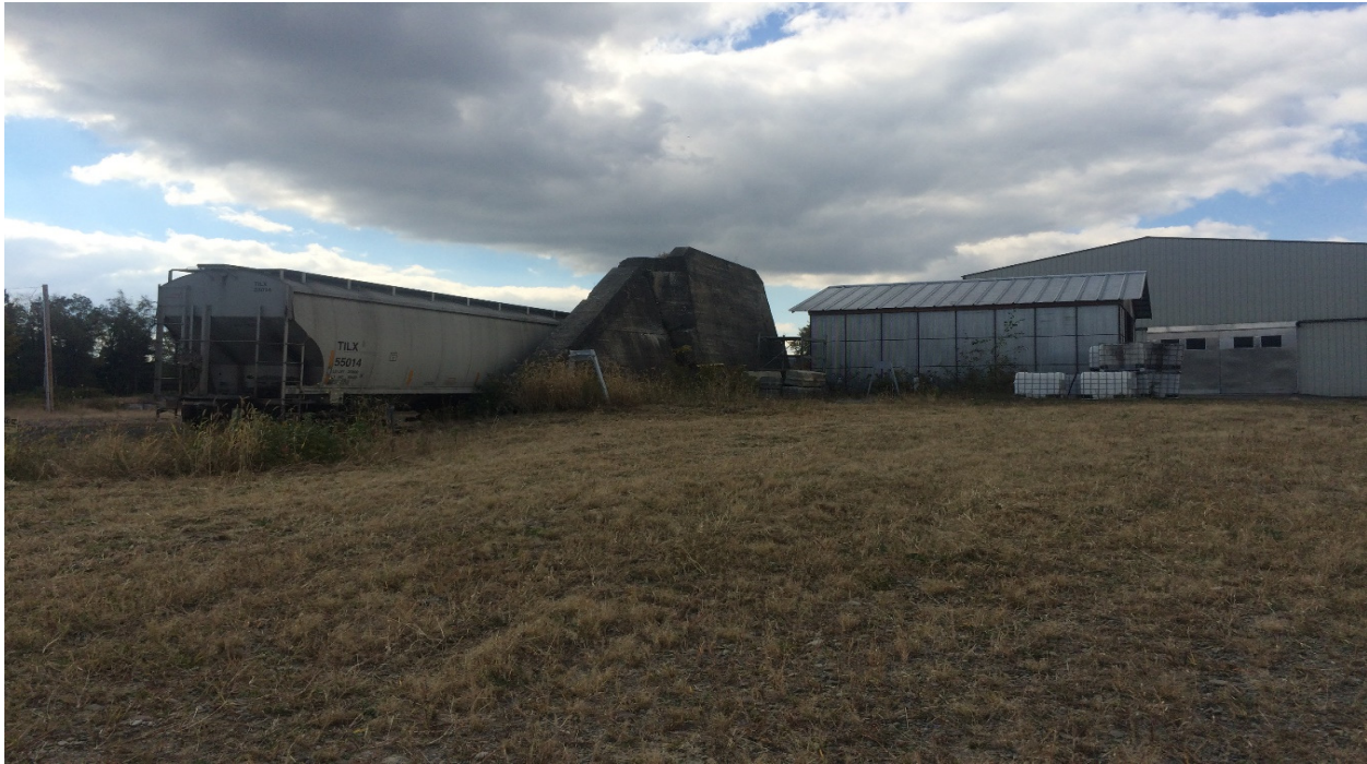
Roundhouse Rd near intersection of Ceperley Ave looking southwesterly toward existing bridge abutment.
