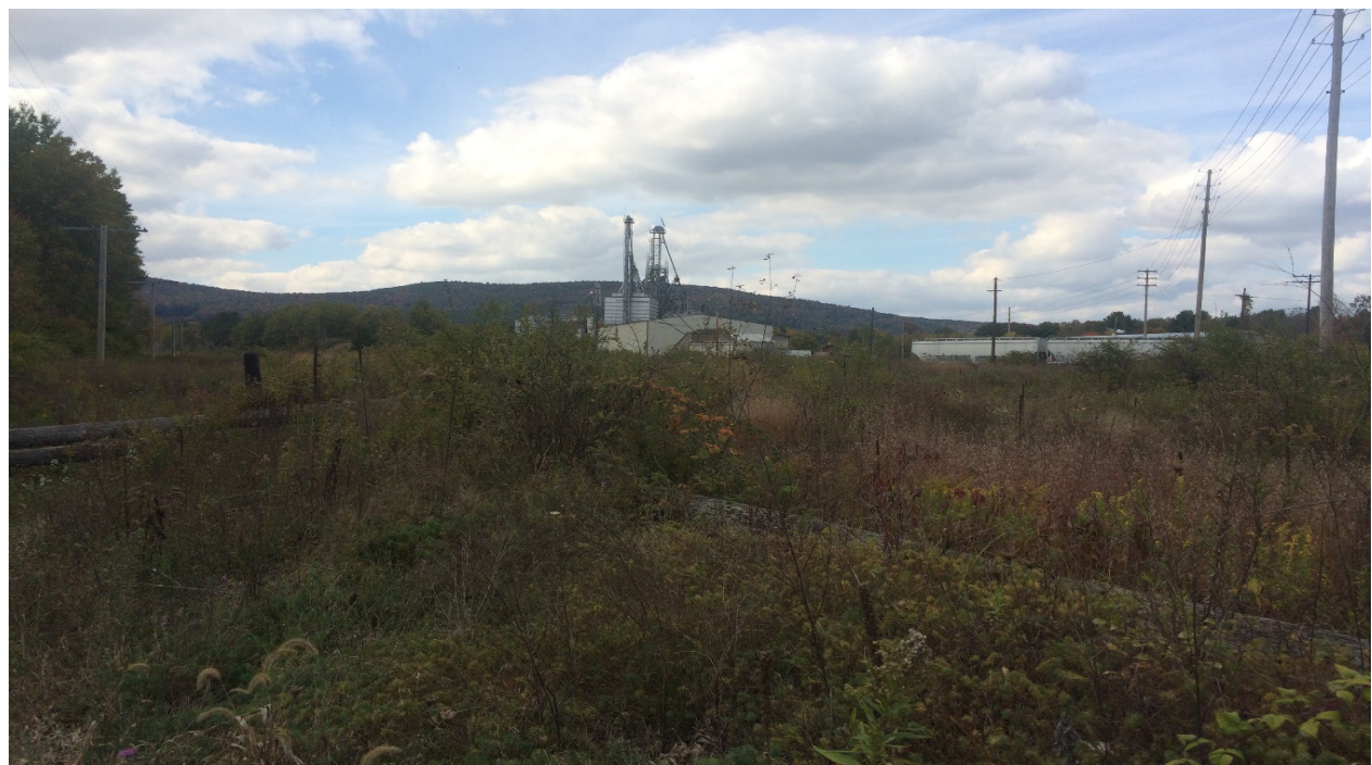
End of River St looking across Railyard at Lutz Feed, Inc.
